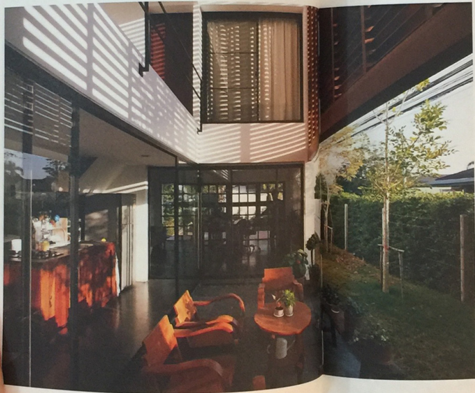
The louvers inside help to shield the outdoor terrace from the mid-day sun.
